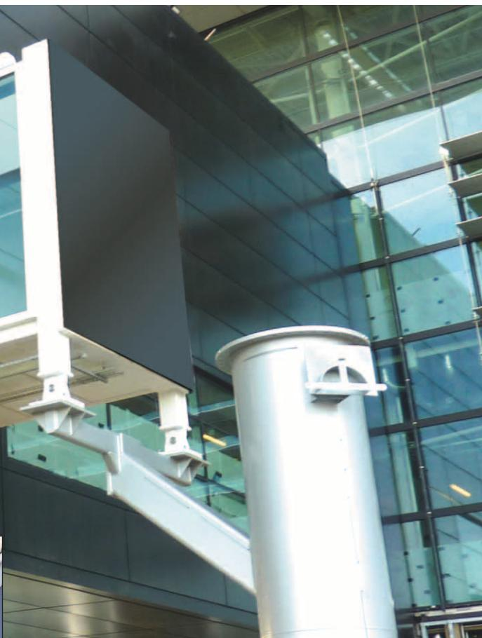
**AirLinks** have been designed in accordance with Eurocodes BS EN 1990, 1991 and 1993, and CE marked in compliance with BE EN 1090.
