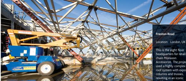
headquarters for retail Accessorize. The project used a highly complex roof system with exposed columns and trusses, resulting in an iconic building.
